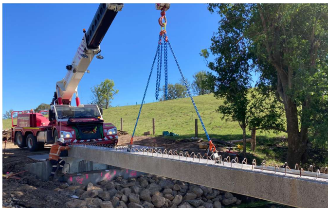
View of Girder Installation at Reeves Bridge by Fortec for Dungog Shire Council
