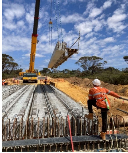
View of Girder Installation at Bridge 5023B by Fortec for MRWA
